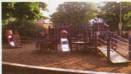
The bark surfacing under the playlot equipment is outdated as it impedes stroller and wheel-chair usage.
